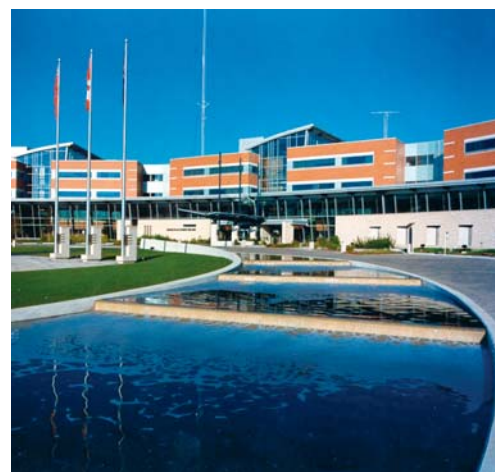
Ontario Provincial Police Headquarters
